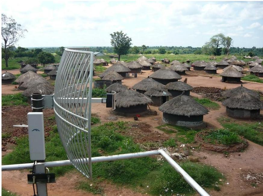
Fig. X: WiFi Antenna attached to a water tower overlooking Coope IDP camp
