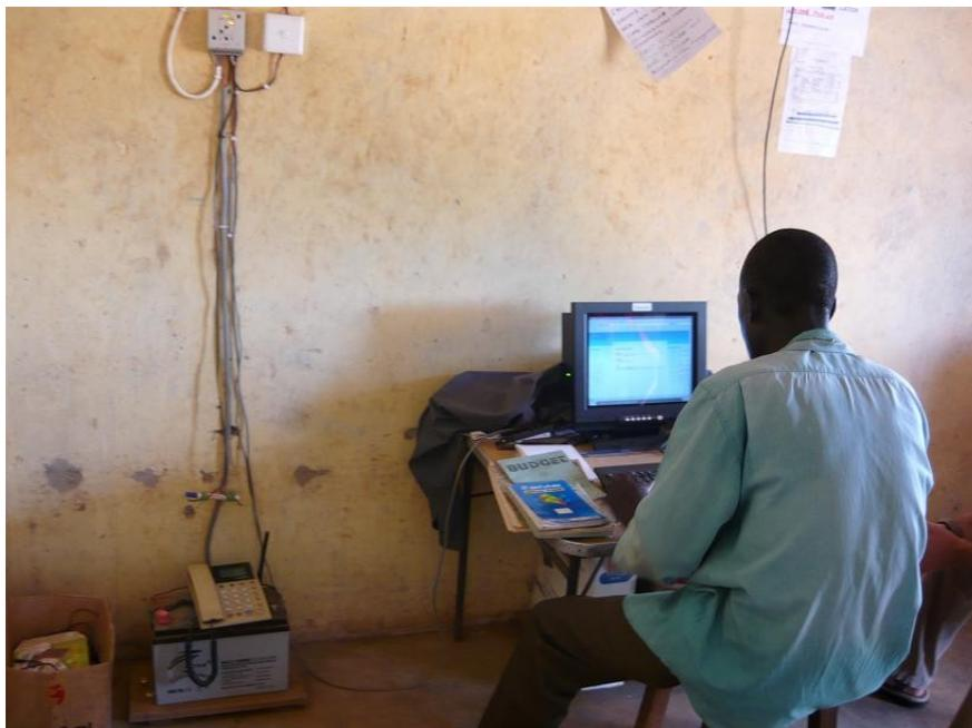
Fig.X: Coope site manager using BOSCO’s wikispace on an Inveneo computer power by a solar charged battery and connected to the WiFi Antenna.
